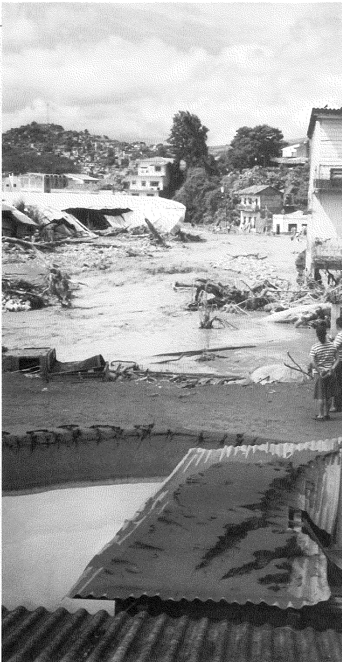
Left: Damaged houses and buildings in Tegucigalpa
