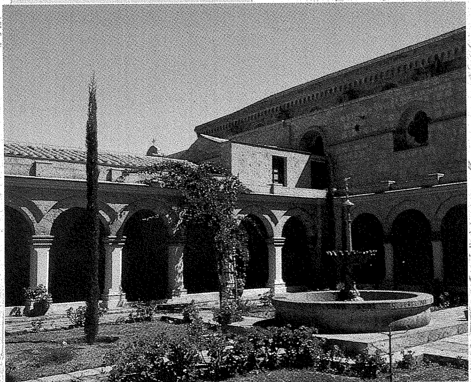
Courtyard of a seminary, also dating from the early eighteenth century, in Arequipa, Peru.
