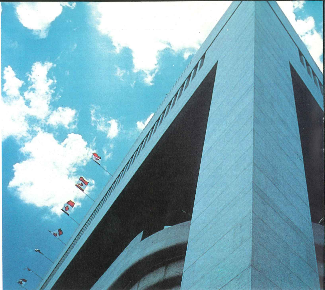
The east corner of the Embassy, reminiscent of a ship's prow, points towards the National Gallery of Art's east wing and the Capitol buildings.
