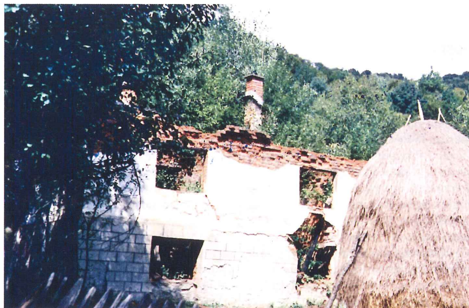
Gutted farmhouse with haystack.
